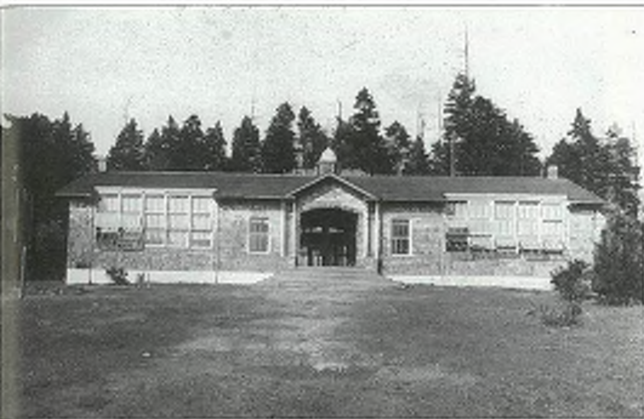
This is the third Rolling Bay School located on "School Hill." It was eventually abandoned in 1929 and demolished in 1941.
